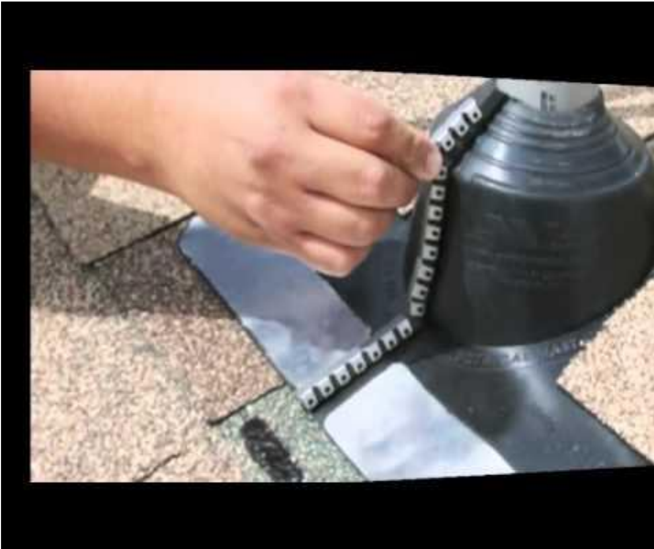
Clips installed over the seam
